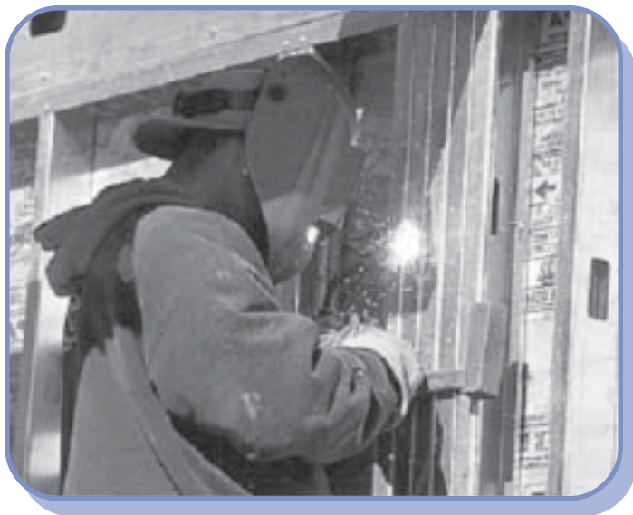
Figure 4.12–Welding of Cold-Formed Steel Framing
